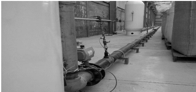
Figure 6. General overview of the test facility.
